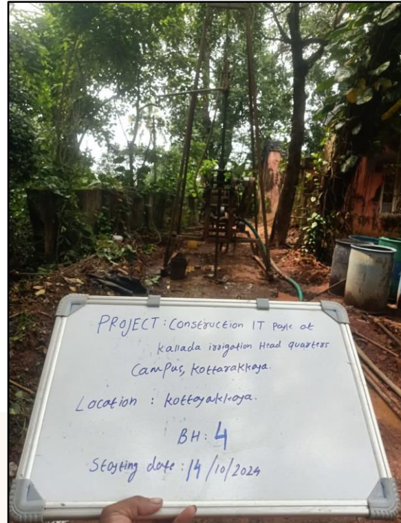
Figure 4: Borehole location at BH-04
