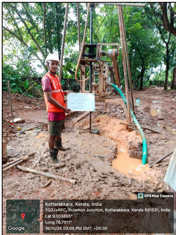
Figure 5: Borehole location at BH-05
