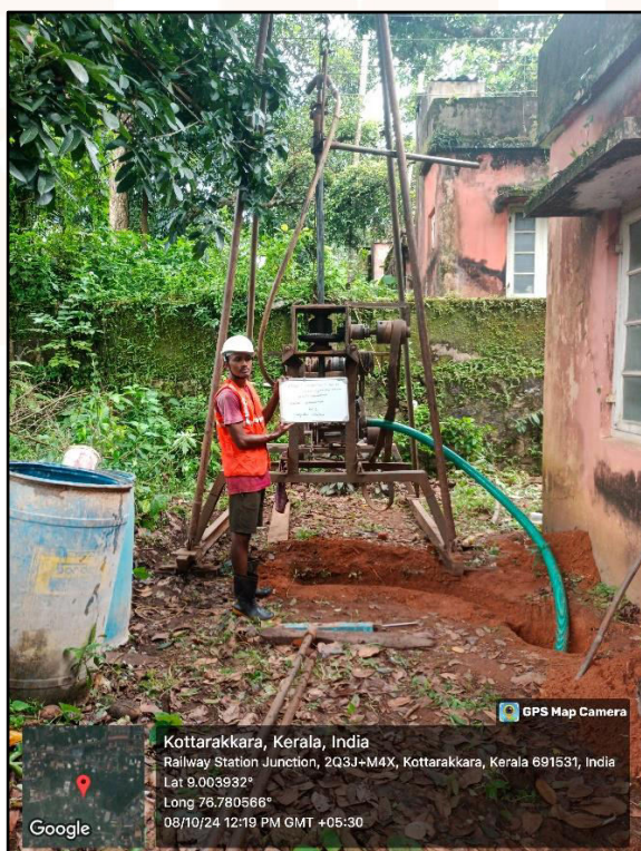
Figure 2: Borehole location at BH-01
