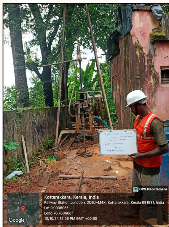
Figure 3: Borehole location at BH-02
