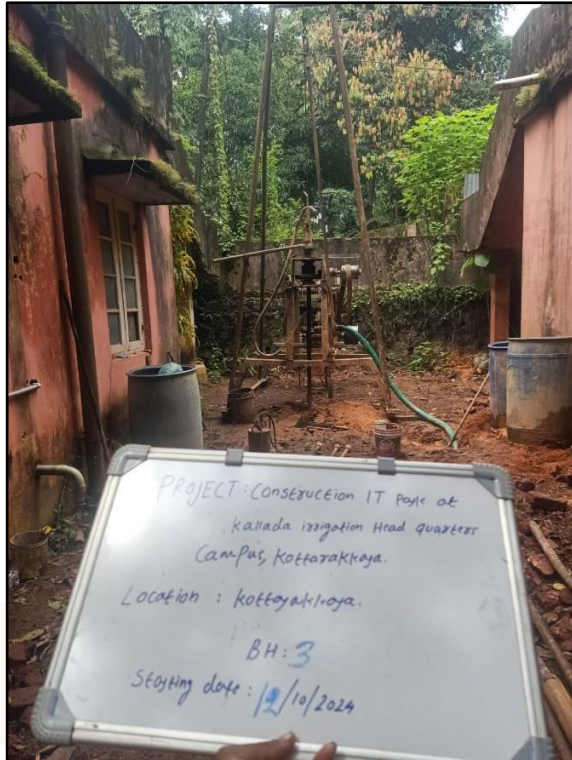
Figure 3: Borehole location at BH-03
