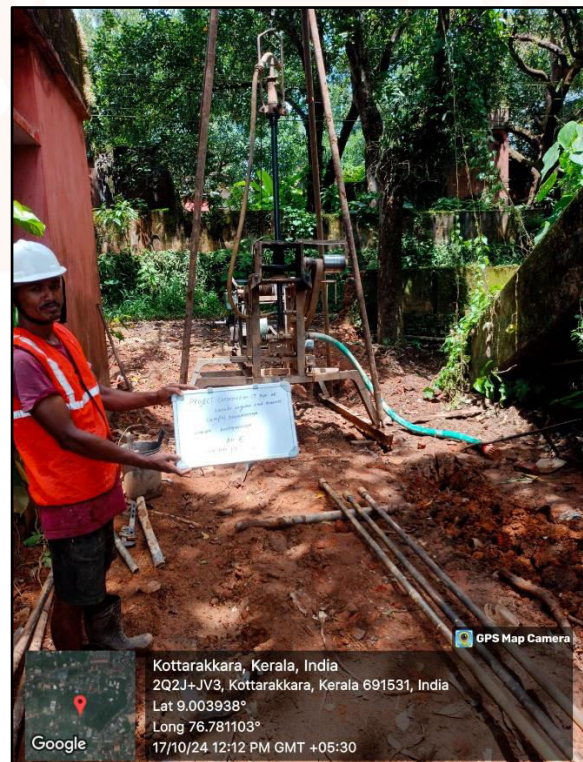
Figure 6: Borehole location at BH-06
